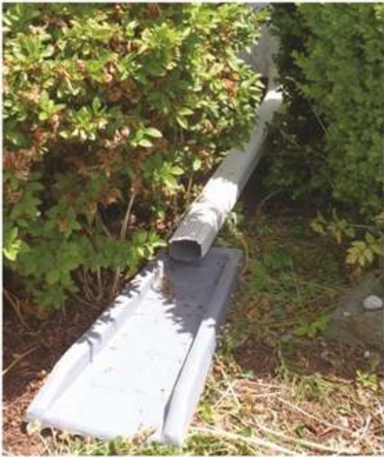
Disconnected downspout
