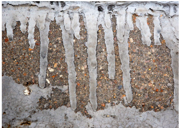
Figure 1: Exterior caulking—a common source of PCBs—used on masonry concrete as a sealant. Photo credit: Steve Snodgrass on Flickr.
