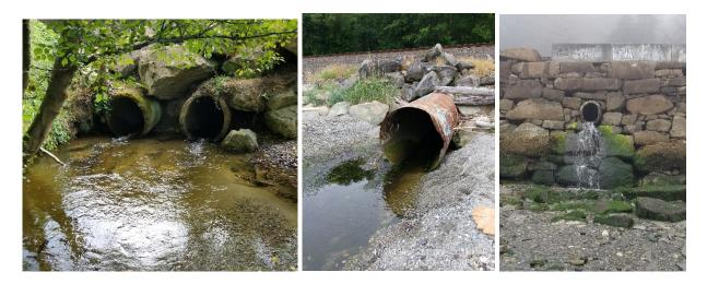
Figure 4. Examples of round culverts encountered in field survey—dual concrete (left), metal (center), concrete (right)
