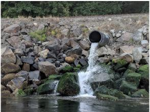
Figure 6. Examples of stream culverts that are at grade (left) and perched (right)
