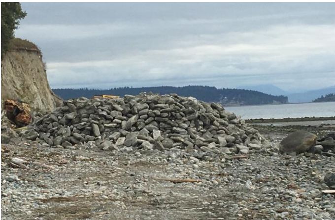
Concrete pillows staged for removal
