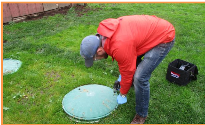
Professional septic inspection in progress.
