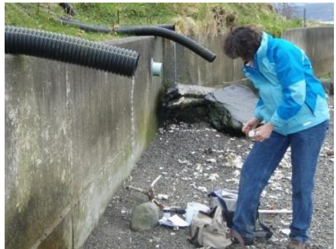
HCRPIC Program team member inspects a shoreline drainpipe. Photo by: Kitsap Public Health District
